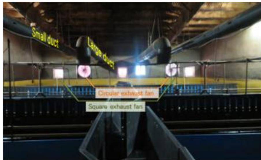
**Figure 1.** Experimental pigpen with mechanical ventilation systems including five different exhaust fans and duct inlets.
