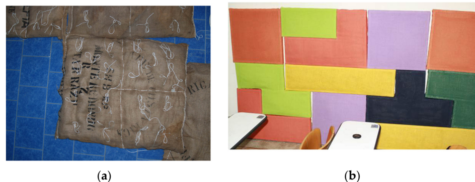
Figure 1. Jute envelopes wrapping the absorption panels (a) and application of absorption coefficients in classrooms (b).
