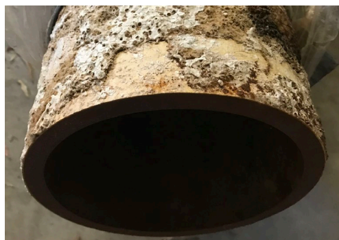
Figure 1. Calcareous deposition on exterior protective coating of a steel pipeline (200 mm (nom.) diam.) with sacrificial anode-protection after 8 years continuous exposure in 10 °C offshore natural seawater (copyright R.E. Melchers).
