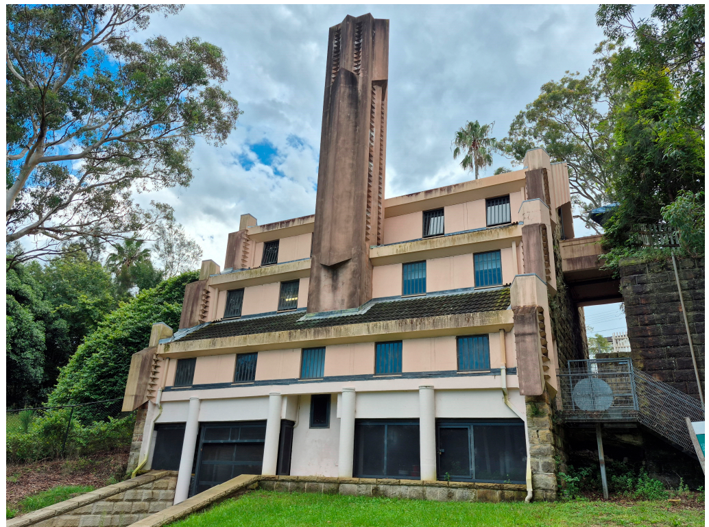
Figure 2. Reverberatory incinerator (NSW039), Willoughby NSW, now operating as a community art space and cafe (Photo: M Parker 2026).
