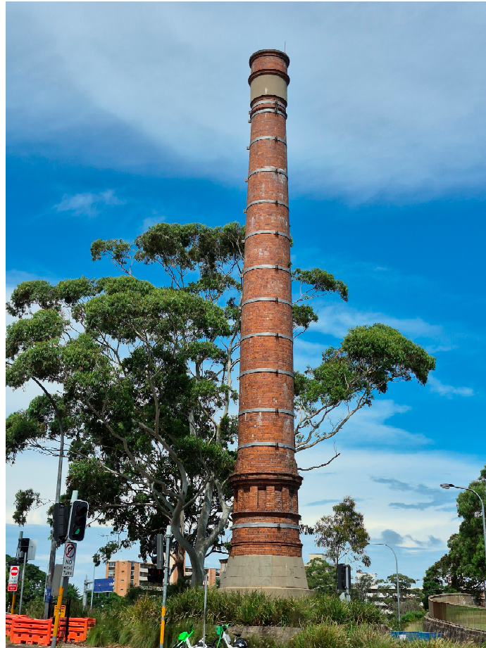
Figure 1. Sewer vent (NSW064 SHR_01641), St Leonards NSW. Part of the original North Sydney sewerage system built between 1891 and 1898 and still operating to mitigate offensive smell emanation from the sewer network (Photo: M Parker 2026).
