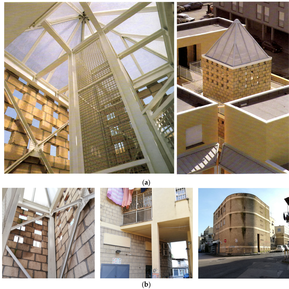
Figure 10. A comparison between (a) Purini and Thermes' completed project and (b) the current state. Closure of the loggias and the deterioration of the tuff facings of the staircases and the front building. (Source: (a) "Controspazio", n. 3 November–December 1988 (b) Photo credit A. Malafronte, 2020).
