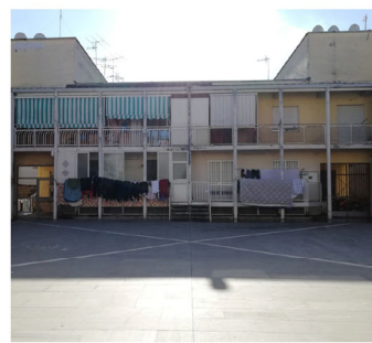
Figure 8. A comparison between (a) Purini and Thermes' completed project and (b) the current state. Closure of the balconies by residents, with consequent alterations to the façade, the construction of volumes not originally planned, improper use of the balconies, and construction of a structure altering the building's crown (Source: (a) "Controspazio", n. 3 Nov.–Dec. 1988 (b) photo credit A. Malafrente, 2020).
