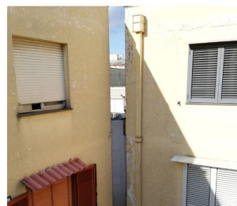
Figure 9. The current state. Alteration of the windows with the addition of projections on the façade and closure of the internal passages between the courtyards and the surface deterioration (Photo credit A. Malafrente, 2020).
