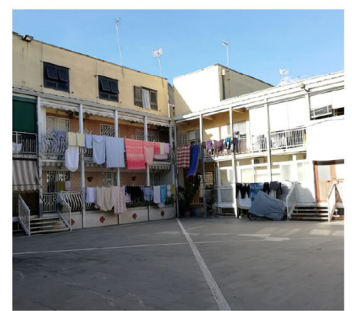
Figure 8. A comparison between (a) Purini and Thermes' completed project and (b) the current state. Closure of the balconies by residents, with consequent alterations to the façade, the construction of volumes not originally planned, improper use of the balconies, and construction of a structure altering the building's crown (Source: (a) "Controspazio", n. 3 Nov.–Dec. 1988 (b) photo credit A. Malafrente, 2020).
