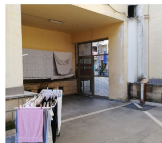
Figure 9. The current state. Alteration of the windows with the addition of projections on the façade and closure of the internal passages between the courtyards and the surface deterioration (Photo credit A. Malafrente, 2020).
