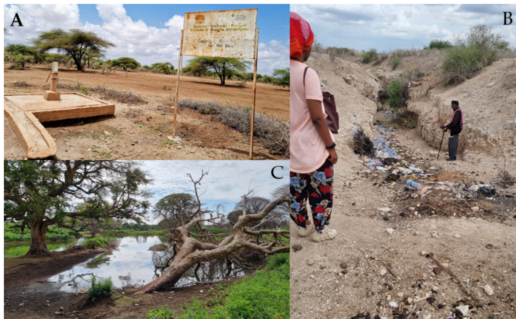
Figure 11. (A) Abandoned modern borehole well, Gayo, Ethiopia, April 2022; (B) litter-strewn abandoned well at Wachille, Ethiopia, April 2024; (C) flooded well, Dubluq, Ethiopia, April 2024 (photo credit: Freda Nkirote M'Mbogori).
