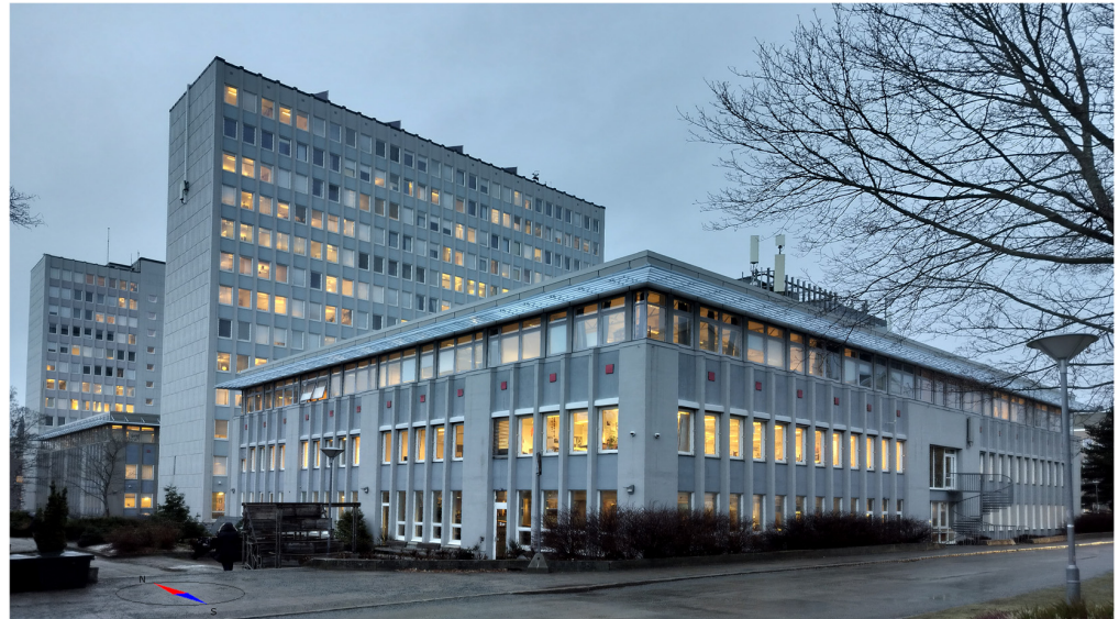
Figure 2. Image of the case study: the central buildings on the NTNU campus Gløshaugen in Trondheim, Norway.
