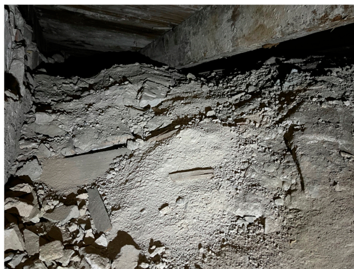
Figure 19. Back of the vault of the Más Palace. Source: Author's own work.
