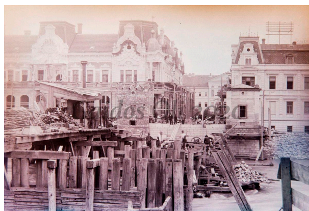
Figure 6. Old photo from the construction of the iron bridge; the old wood bridge can be observed and the customs houses [26].
