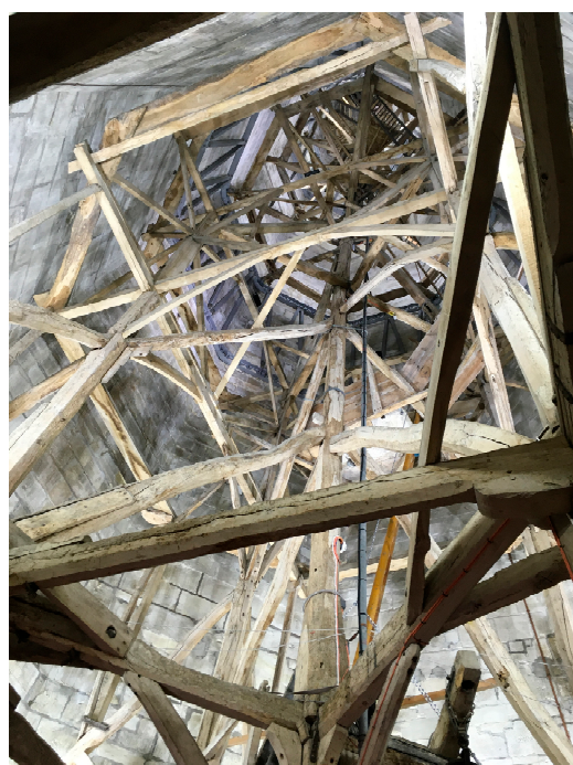
Figure 22. The scaffold inside the Salisbury spire. Source: author's photo.
