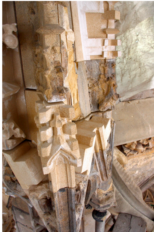
Figure 6. On-site restoration work on a pinnacle at the Stephanskirche, Vienna. It can be observed on the replaced pieces that, first, the geometrical base shape of the details is carved, similarly to the 3D model in this article. Source: author's photo, 2013.
