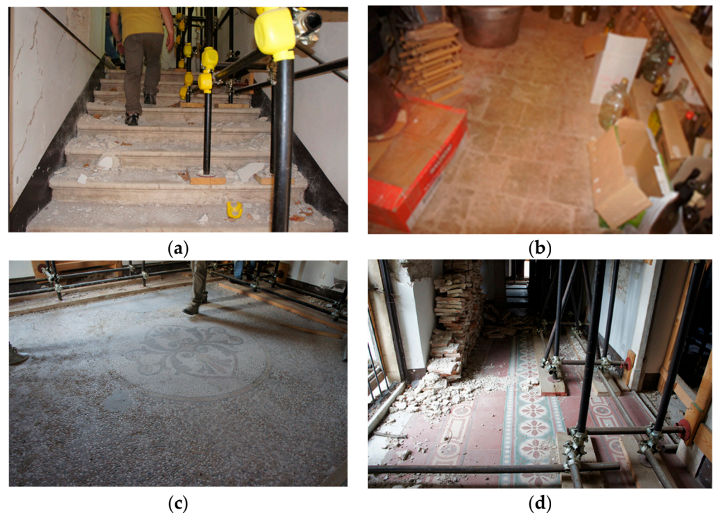
Figure 6. Palazzo Galeota. Photos of the interior details: (a) stone staircase; (b) terracotta floor; (c) Venetian floor; (d) concrete tile floor.
