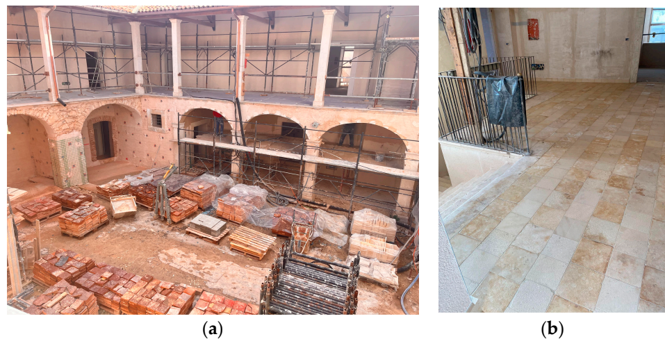
Figure 9. Palazzo Galeota: (a) stacking reclaimed material in the inner courtyard of the building; (b) application of salvaged material in paving stone basalt paving.
