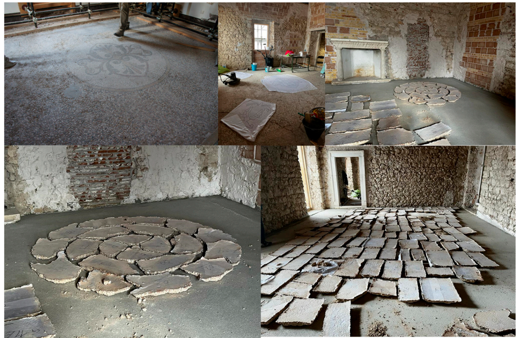
Figure 10. Palazzo Galeota. Work effected on Venetian mosaic floor. From the top left, steps of removal, cataloguing, cleaning and future reinstallation on consolidated vault equipped with radiant floor panels.
