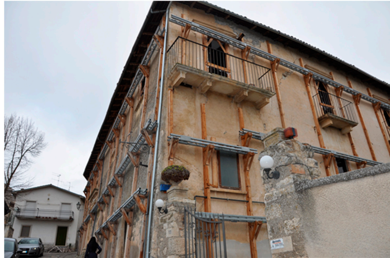
Figure 5. Corner of facade of “palazzo Galeota” facing Galeota Street. Post-earthquake 2009 provisional systems are present on the facade.
