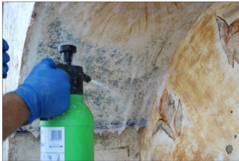
Figure 15. Nebulization of the biocide.
