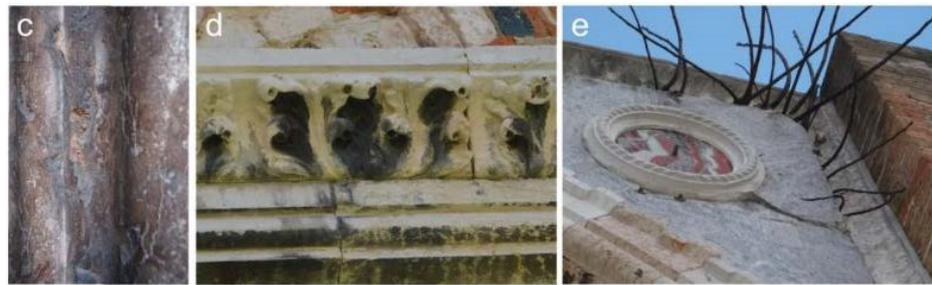
**Figure 1.** Details of the main façade of the ruins of Santa Maria dei Servi Church: (a) the external main portal; (b) the internal main portal; (c) exfoliation of red Verona marble used in the portal; (d) detail of ornamental Istrian stone use in the portal with black crusts in sheltered areas; (e) detail with Proconnesian marble (grey) and the *tondo* in *Cipollino marble* (red); secondary plants (*figus carica*) growth is also visible.
