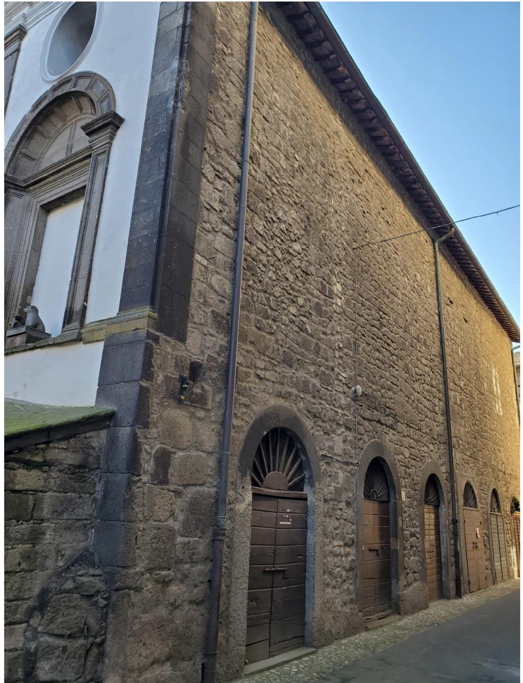
**Figure 7.** The barrel vaults system supporting the right lateral nave of the church. This system is the only one visible from the exterior and is also partially detectable in the GPR results in Figure 6. Based on the GPR results beneath the left lateral nave, it is presumed that the same structural system has been replicated.
