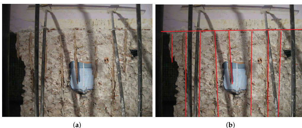
Figure 4. Typology No. 2 in the second floor of Aggregato n.10, Casino Branconio. The T-F wall bears a masonry barrel vault. The narrow-spaced timber posts isolate slender masonry elements, see (a). The red lines in (b) mark the position of the timber posts.
