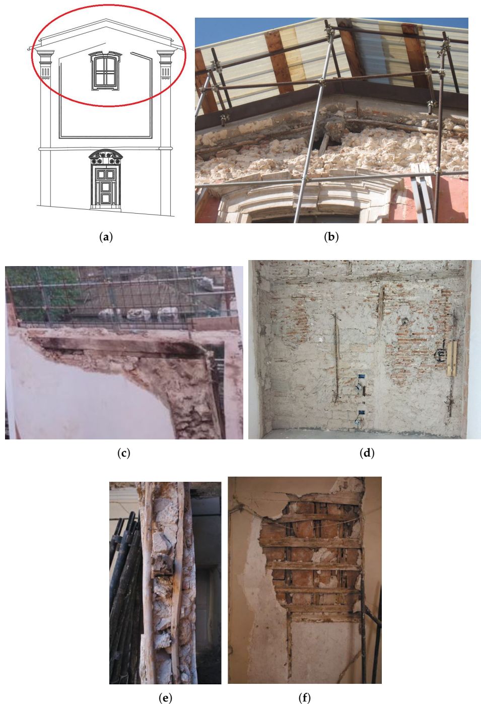
Figure 8. Typology no.6 baraccato . This class gathers all T-F masonry samples, which are challenging to classify; (b,c) T-F structure embedded in the upper tympanum of a church. The tympanum experienced substantial out-of-plane damages from the 2009 earthquake. (c) Timber tie running around the upper part of a masonry wall. (d) Widespread T-F structure without singular regularity, picture from Aggregato no.3. (e,f) Samples of some partition walls found in Palazzo Ardinghelli, Aggregato n.13; The distinction from typology no.1 attains the use of narrow-spaced horizontal posts, yielding a sort of opus cratitium .
