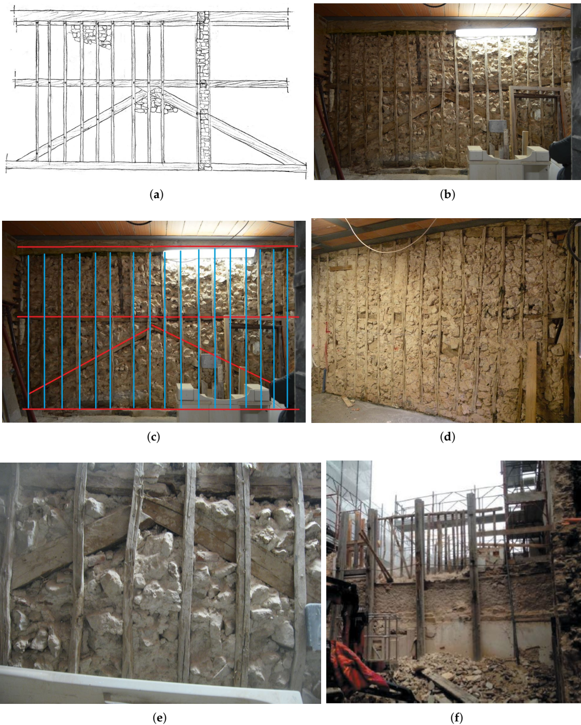
Figure 5. Typology no.3 baraccato in Aggregato n.6. (a) presents a picture of this structure depicting the vertical timber posts fastened to upper, middle and lower horizontal bracings, the diagonal bracings and the included masonry. (b–d) front and rear of the masonry panel. (e) View over the V-type bracing's connection. (f) Picture of Aggregato n.6 during the reconstruction works; The masonry was eliminated, thus showing the vertical timber bracings which encompass two levels.
