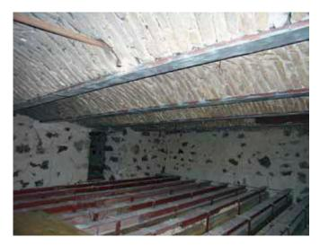
Figure 24. The lowered domes system of the roof of the 2nd floor.
