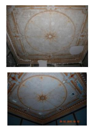
**Figure 39.** Painting decoration of a room ceiling of the 2nd floor before (**top**) and after (**bottom**) the restoration works (2015).
