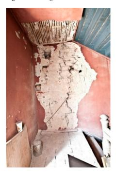
Figure 27. Longitudinal cracks in the central stairway area.
