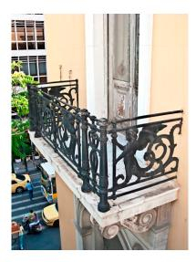
**Figure 10.** Balcony of the 2nd floor with the cast iron railings and the marble beads (2009). C.S.J.S.F. Photographic Archive.
