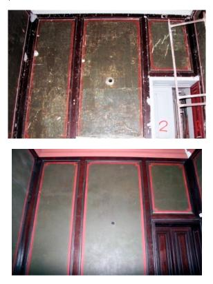
**Figure 38.** Painting decoration of walls of the 1st floor before (**top**) and after (**bottom**) the restoration works (2015).
