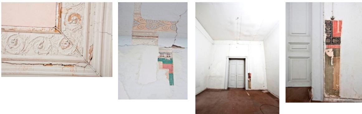
**Figure 29.** Covering of painting layers on ceilings and walls of the 1st and 2nd floor.
