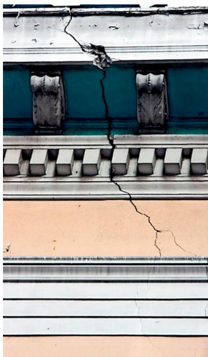
**Figure 25.** Naturally caused changes by earthquakes.
