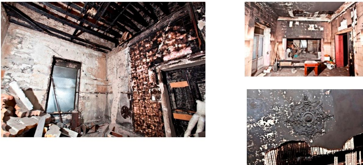
**Figure 30.** Damages due to the 1996 fire on the 2nd floor.
