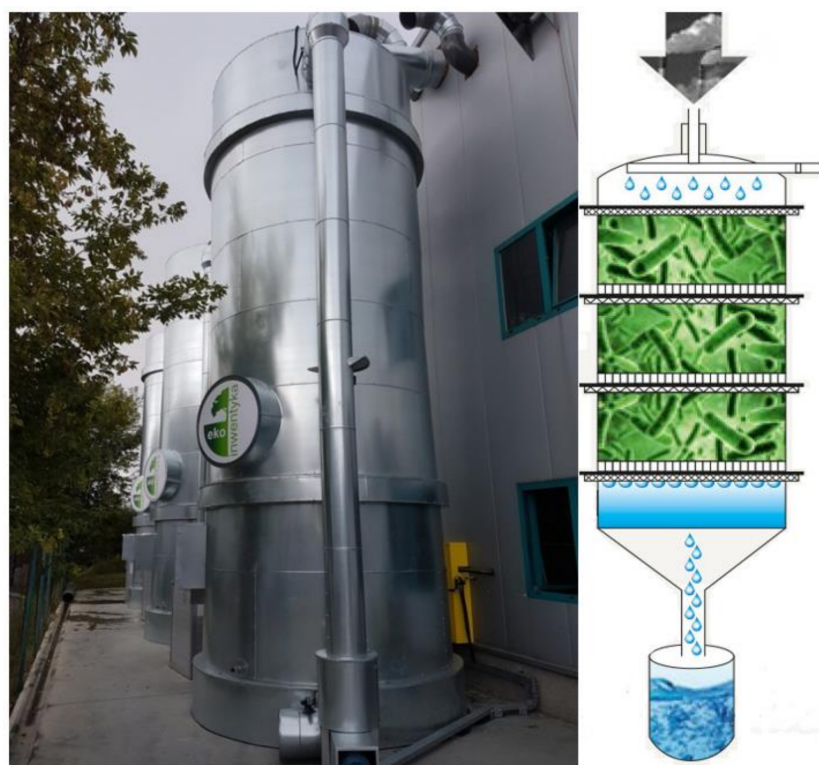
Figure 5. Compact Trickle Bed Bioreactors in full industrial scale (Compact Trickle Bed Bioreactors, Manufacturer: Ekoinwentyka LTD, Ruda Śląska, Poland), Reproduced from [54], Industrial varnishing: 2020.
