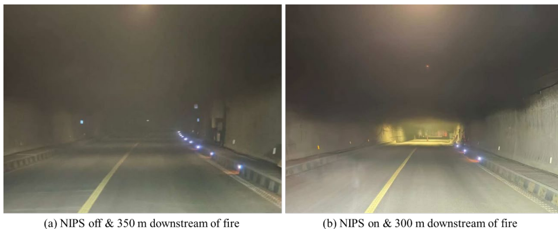
Figure 18. Smoke distribution downstream of the fire source under fire conditions in the full-scale tunnel.
