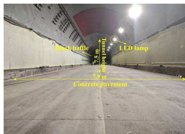
Figure 4. Internal view of test tunnel.
