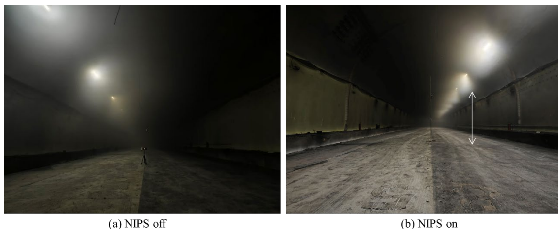
Figure 14. Smoke distribution in the downstream tunnel section 15 min after ignition.
