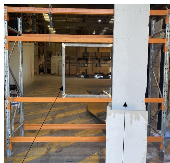
L-angle frame to hold the window glass
