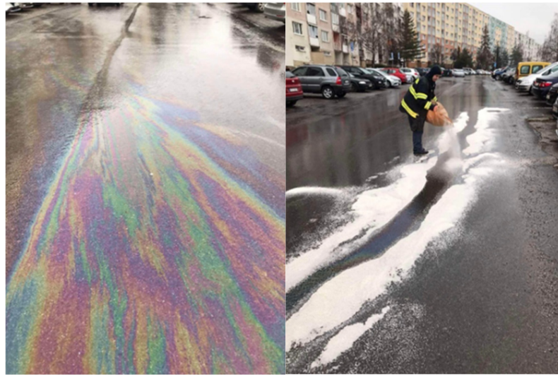
Figure 18. Leaked operating fluids on the road and their backfilling using sorbents (source: elaborated by authors).
