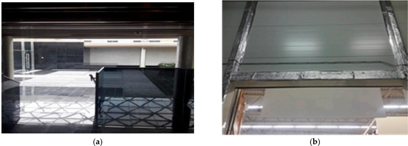
**Figure 1.** Fire curtain in: (a) Public space of an apartment complex; (b) Shopping mall.
