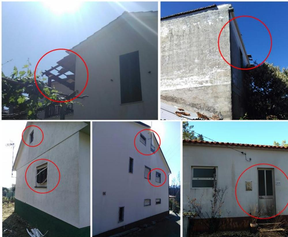
**Figure 6.** Details of some elements that were damaged by the fire but with no ignition to the house.
