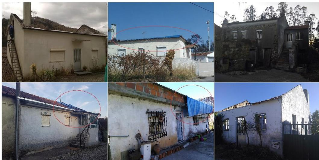
**Figure 7.** Example of houses that had ignitions through the roof.
