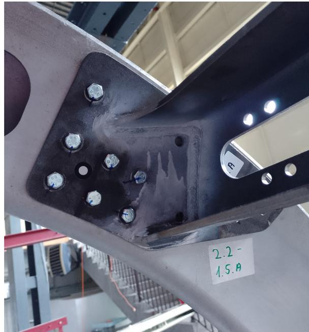
**Figure 8.** Bolt and screws verification.
