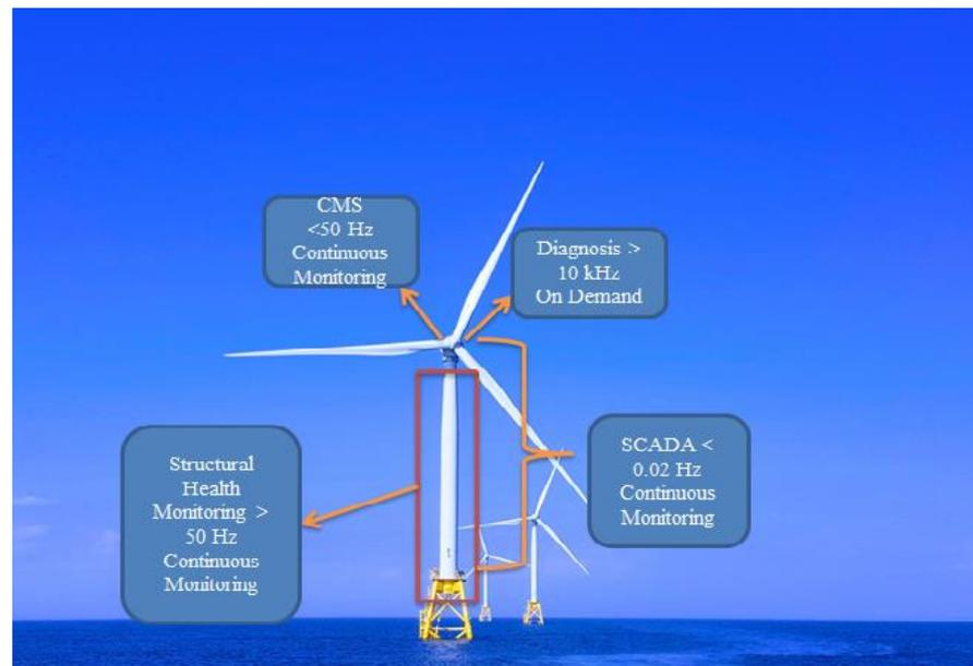
**Figure 15.** SCADA and CMS systems common description and specifications of use.
