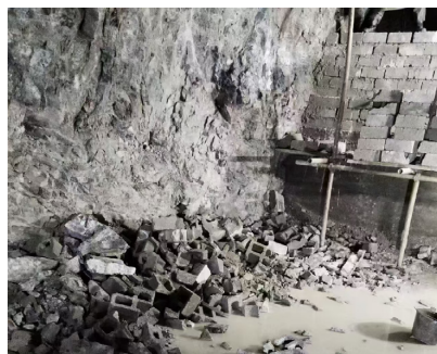
Figure 2. Filling Retaining Wall No. 34N.
