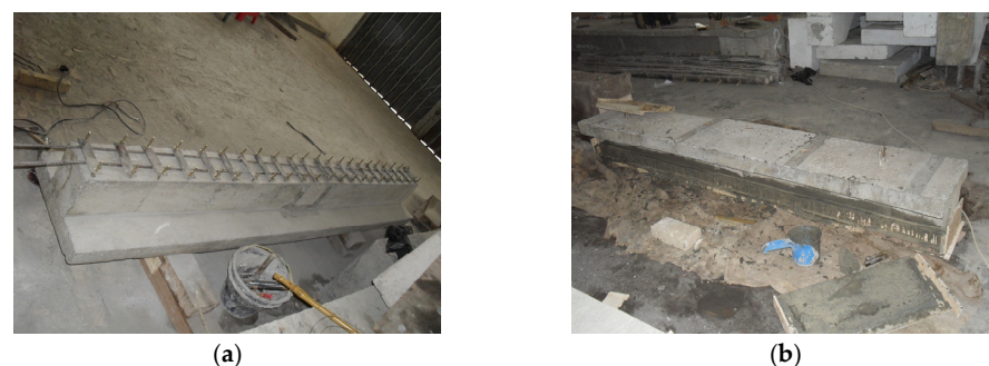
Figure 2. Installation of the SWR strengthening system: (a) anchoring of SWRs using steel plates and dynabolts; (b) application of the mortar adhesive.
