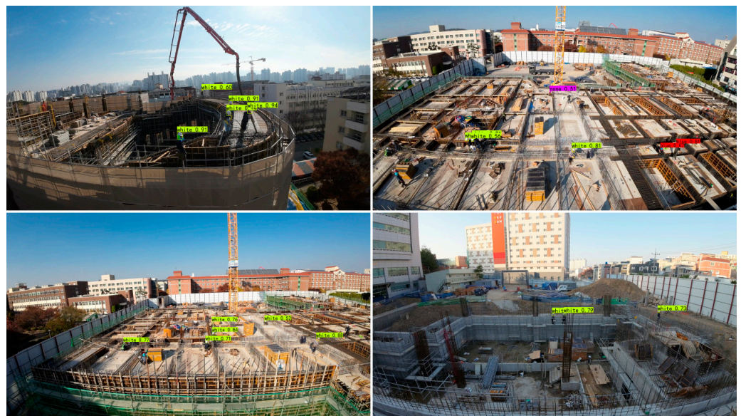
Figure 7. The visualization results of Liang et al.'s proposed automated detection method for helmeted workers using UAVs on construction sites [111].
