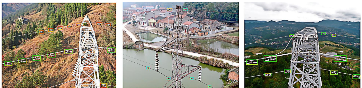
Figure 14. Experimental results of the PMA-YOLO network for the detection of anomalous vibration dampers [57]. The ground truth boxes and prediction boxes for “rusty”, “defective”, and “normal” dampers are shown in yellow, red, blue, and green, respectively.
