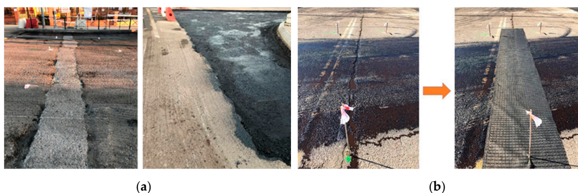
Figure 2. (a) Discontinuities in urban roads; (b) Incorrect performance over a longitudinal cracking.
