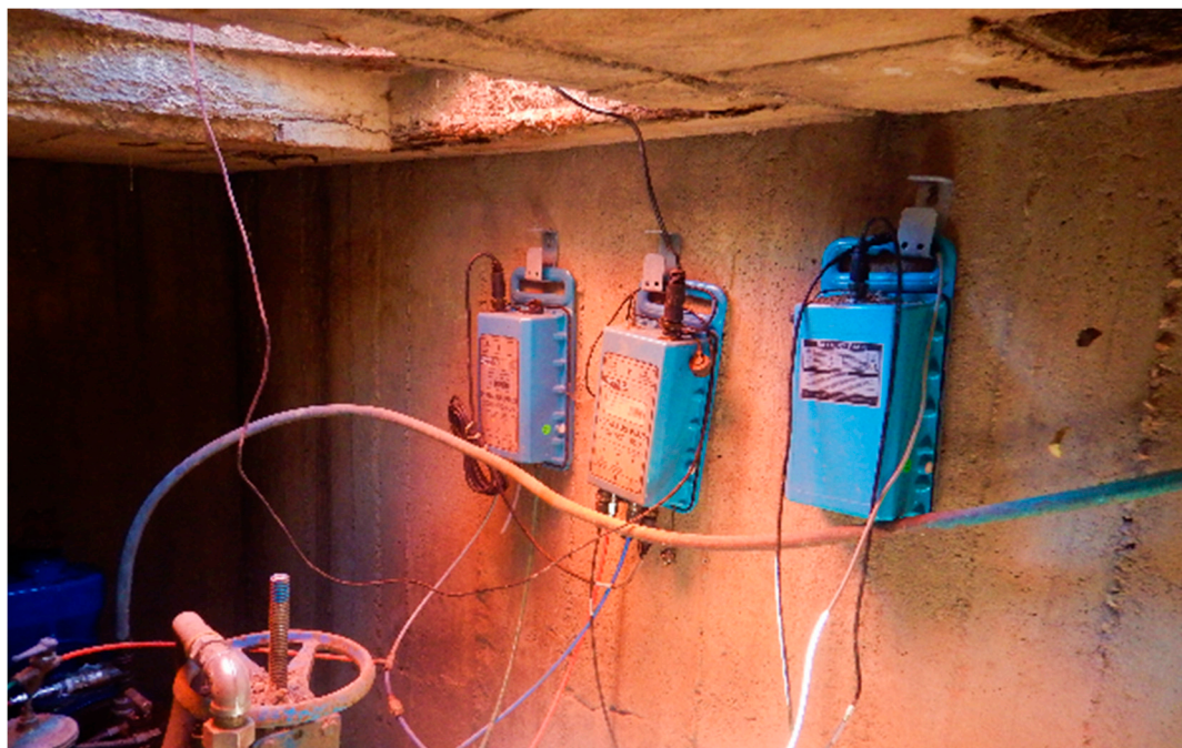
Figure 2. The Pegasus+ controller at the PRV installation site.
