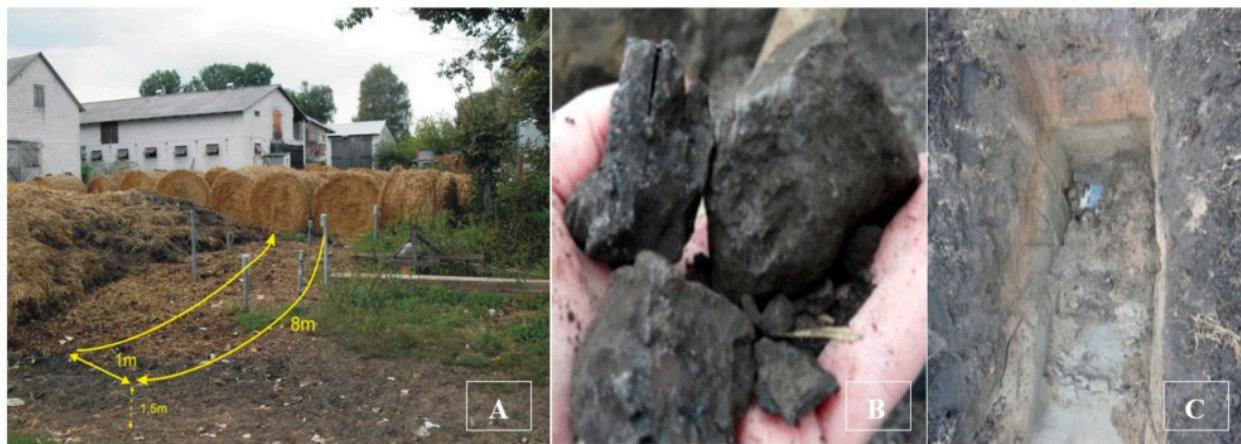
Figure 2. Constructed vertical deposit of permeable organic barrier in the leachate flow path from unprotected storage manure in a cow farm (photo S. Szklarek, J. Wójcik). (A)—vertical deposit of the permeable organic barrier with pipe wells for monitoring ground water, (B)—lignite and charcoal lime were used as sources of organic carbon, (C)—ditch 1.3–1.5 m deep and 1 m wide situated perpendicular to the slope/direction of groundwater flow.
