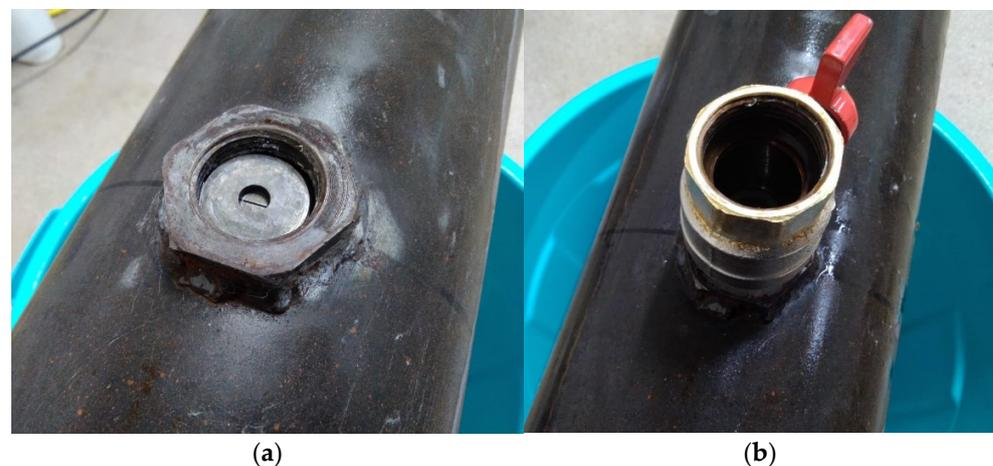
**Figure 4.** The method of mounting discs on the pipe: (a) laying discs; (b) installing a ball valve on top of discs.
