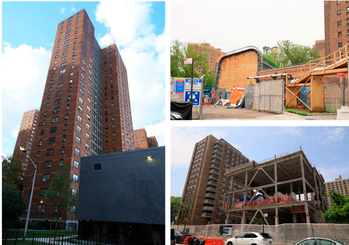
Figure 4. Restoration works as part of Sandy Recovery Program at public housing developments in NYC. Source: Author, 2022.
