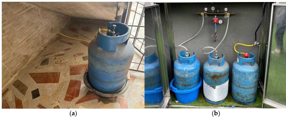
Figure 4. Observed conditions of the cylinders: (a) cylinder showing condensation; (b) cylinder undergoing freezing.
