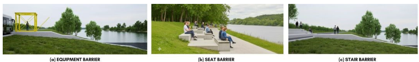
Figure 3. Types of hybrid flood-protection barriers along urban riverfronts: (a) Equipment barrier, where the structure itself (e.g., shelter or stop) functions as a retaining element; (b) Seat barrier, which integrates protection into public furniture; and (c) Stair barrier, which adapts the slope to both protect and connect the urban and fluvial levels.
