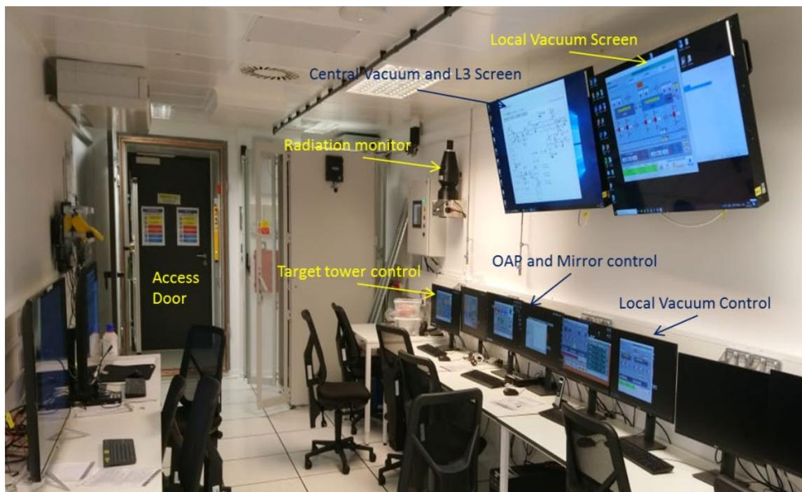
**Figure 1.** Photo of the E4 local control room. The screens show some key control software (central vacuum and mechanics). The dose rate monitor LB 6419 is visible next to the second large screen on the wall. The E4 hall access is interlocked and has EMP shielding. The graphic interfaces for some of the ELIMAIA controls are detailed in the next sections.
