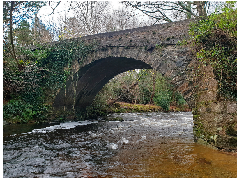
Figure 9. Typical defect photo shows scour to abutments and vegetation cover including trees.
