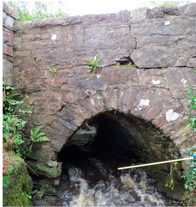
Figure 8. Typical defect photo shows scour to abutments, missing masonry, pointing loss, and cracking.
