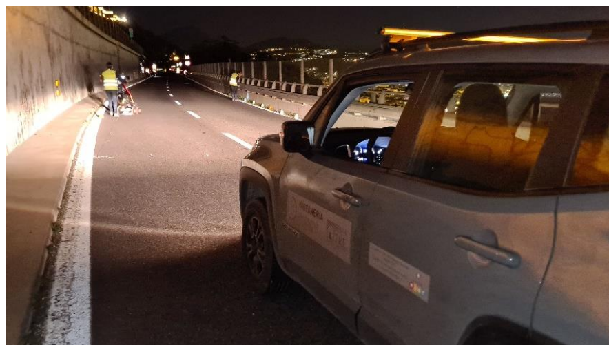
Figure 7. A section of the inspected highway during the survey.
