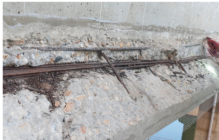
Figure 5. Deterioration of internal tendons in a PSC bridge (2021).
