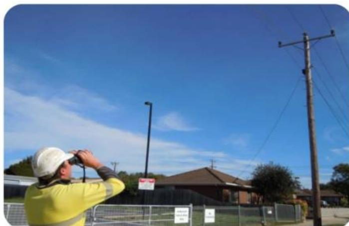
**Figure 3.** Visual inspection technique carried out from ground [16].
