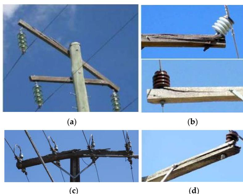
**Figure 1.** Deteriorated and failed timber crossarms due to decay and aeolian vibrations; (a) failed crossarm losing an insulator; (b) splitting at the end bolt locations; (c) badly split crossarm along the length; (d) losing sound wood at the end of the crossarm.
