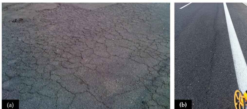
Figure 7. Examples of (a) alligator cracking and (b) longitudinal cracking.
