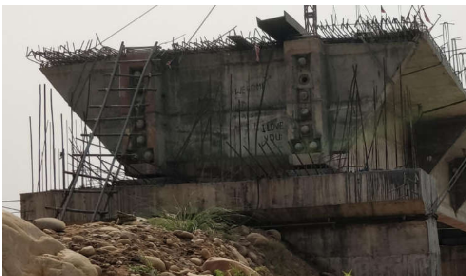
Figure 25. End of Span-4 over Abutment-2. Some temporary suspension cables were anchored at abutment and others were anchored near the end of Span-4 deck.
