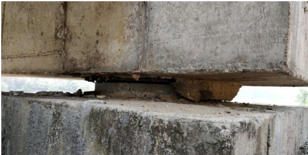
Figure 13. Pot bearing system above Abutment-2 (Undamaged).
