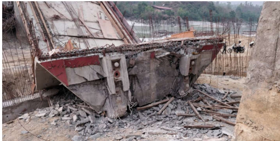
Figure 7. Horizontal shear failure at construction-joint level as the lower part of the beam that included four prestressing ducts slid inwards.
