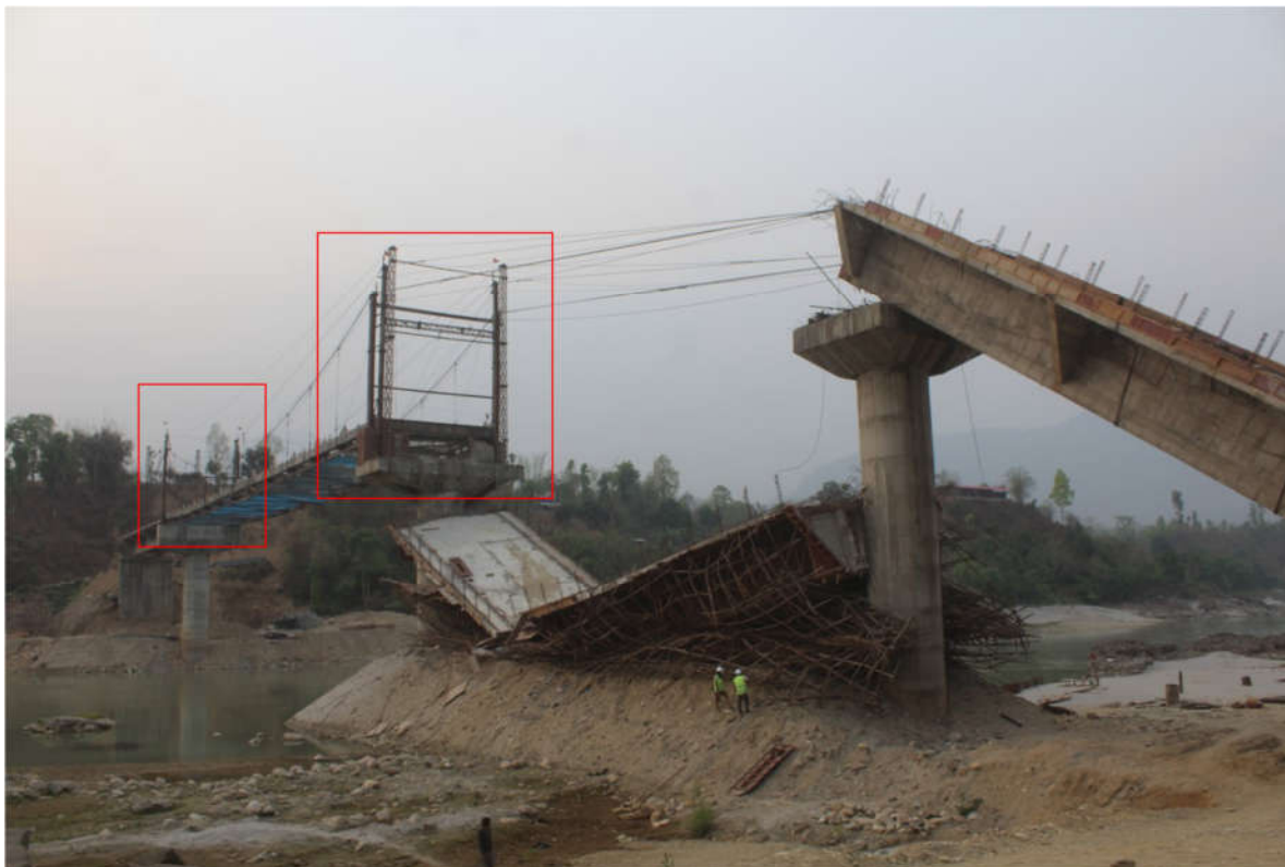
Figure 3. Steel towers constructed on pedestal.
