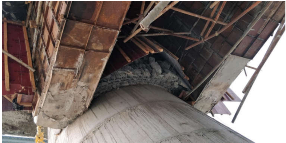
Figure 17. Bearing indentation in the beam with sheared bolts lodged (Pier-2).
