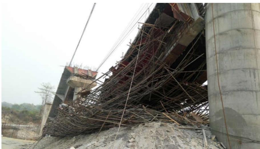
Figure 22. Falsework damage in Span-2; buckling was mostly towards upstream side, indicating damage initiation by settlement of downstream side first.
