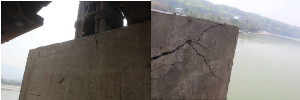
Figure 27. Damage to the RCC pedestal over pier-cap of Pier-2; steel tower was erected over it as a temporary structure for prestressing.
