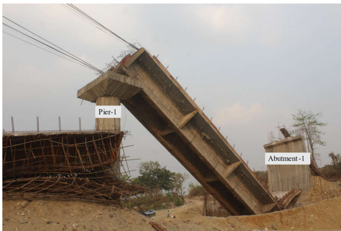
Figure 4. Collapsed first span of the bridge.
