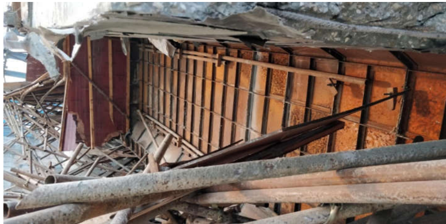
Figure 23. Intact formwork on other part of Span-2 (except the beam fracture location), indicating failure mechanism consists only one failure location.
