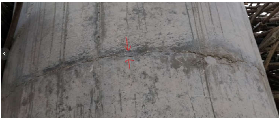
Figure 21. Horizontal crack towards the Span-1 side of Pier-1, at 2.5 m height from the ground level.
