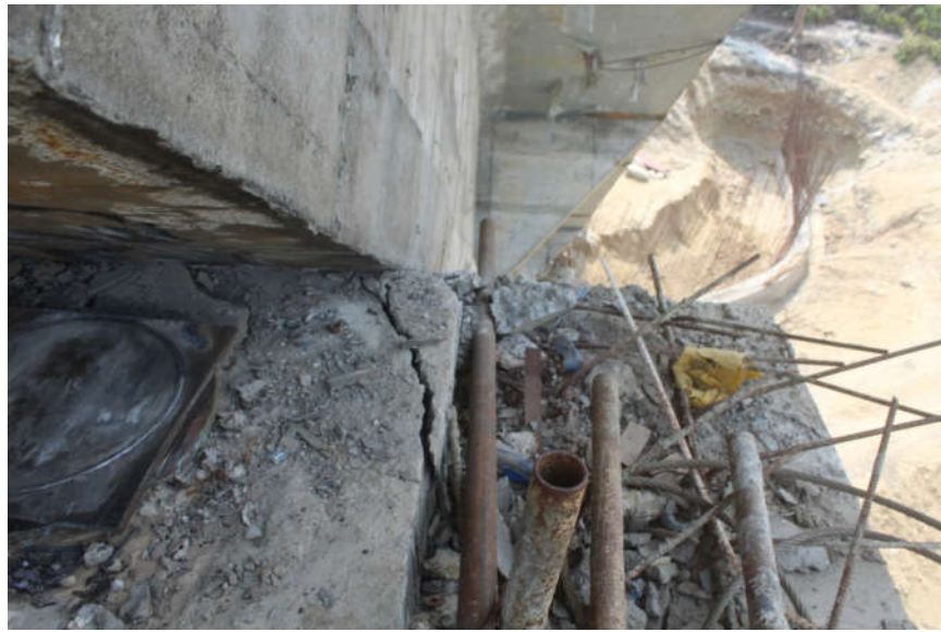
Figure 19. Damage to pier cap of Pier-1 due to Span-1 collapse.
