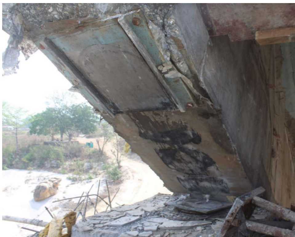
Figure 16. Span-1 deck (over Pier-1) that slid about 1 m towards Pier-1 indicating drag of deck (shown by bearing mark under the beam surface) and damage of bearing.
