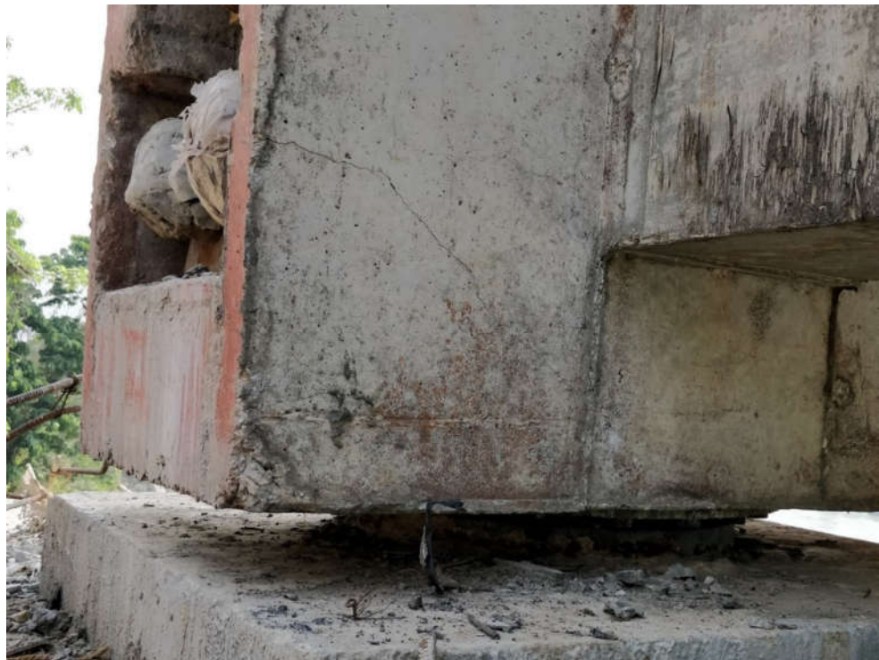
Figure 24. Some cracks around the end of Span-4 lower prestressing cable anchor zone, on Abutment-2 side.
