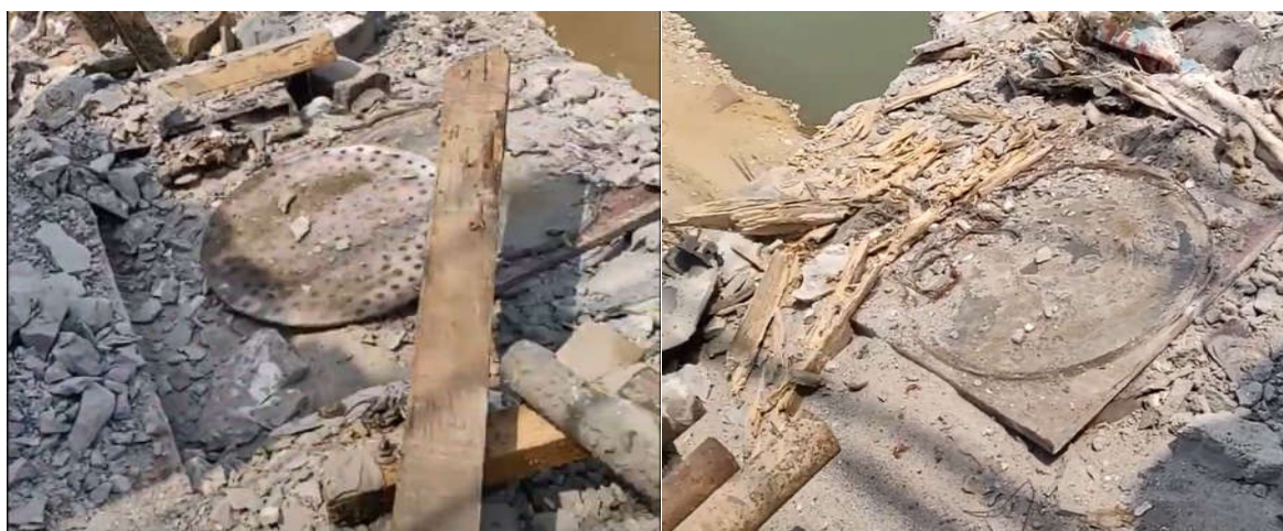
Figure 15. Damaged bearing above Pier-1, span-2 side (downstream and upstream side).
