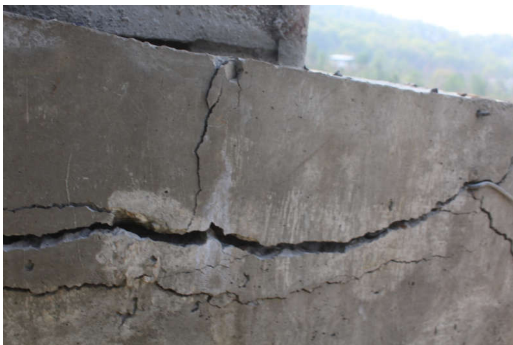
Figure 26. Heavily damaged pier cap above Pier-2 due to the tensile action exerted by the temporary suspension cables on the steel towers.
