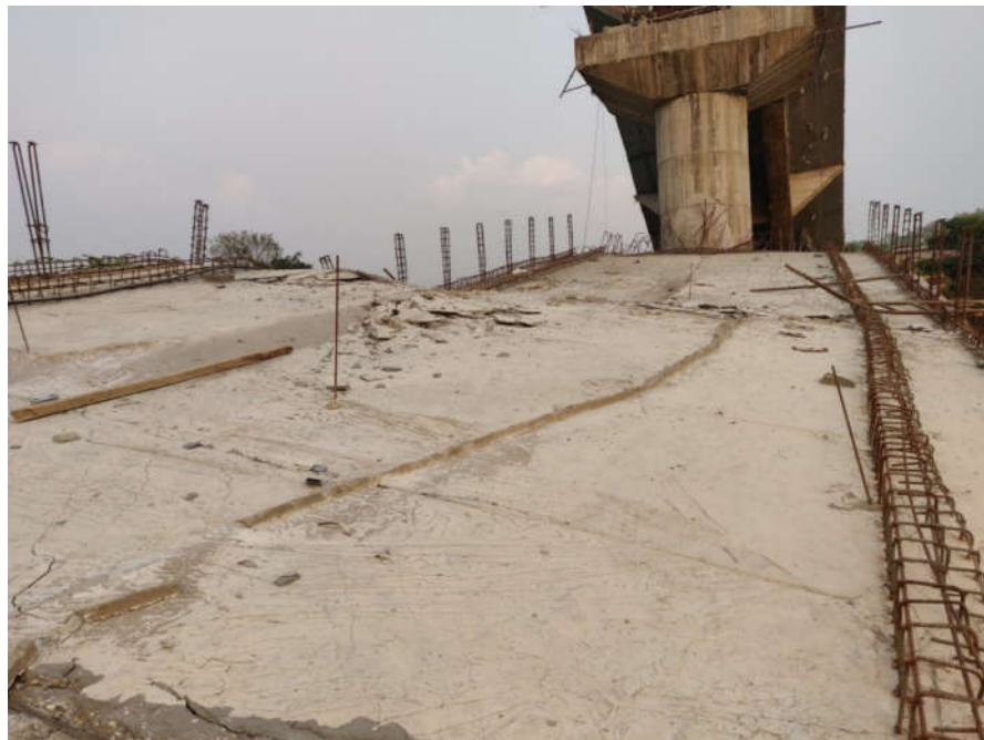
Figure 10. Cracks observed along the slab surface of Span-2.
