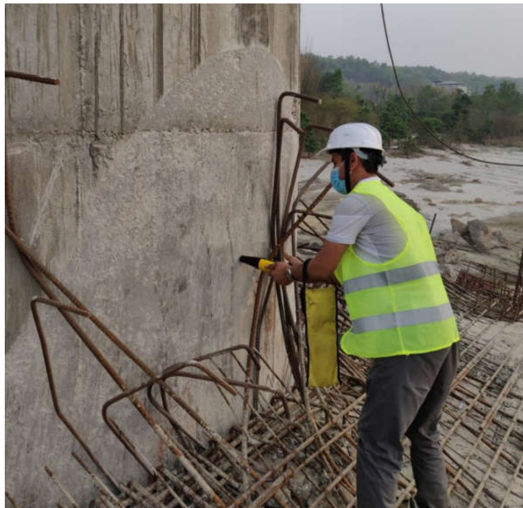
Figure 18. Damage to Pier-1 by end cross beam of Span-2 during collapse.
