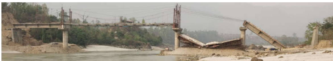
Figure 2. Thimura prestressed bridge with two collapsed spans.
