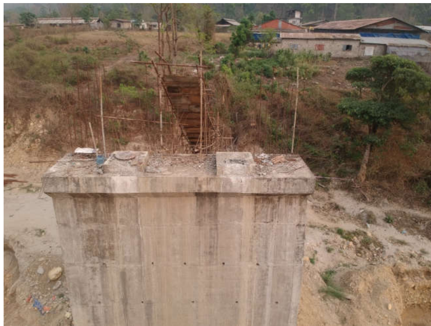
Figure 14. Bearing damage in Abutment-1 due to slippage of the slab before falling.
