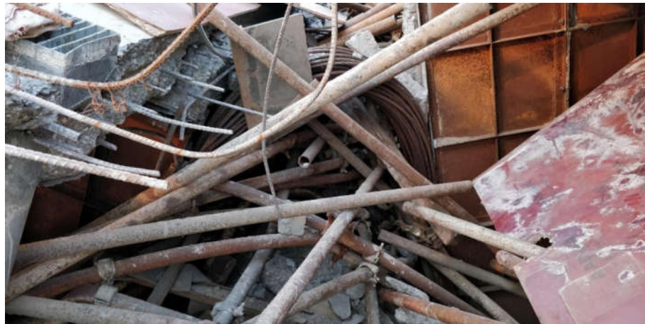
Figure 11. Several bars in the slab of Span-2 can be observed being pulled out and show up in pairs, indicating the significant lapping region of the slab; the prestressing cables were also pulled out to significant length during collapse.
