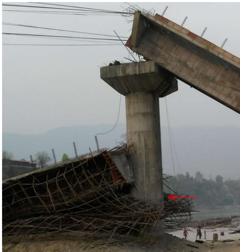
Figure 20. Pier-1 being pushed by Span-1 from the top and Span-2 from the middle in opposite directions. Horizontal crack is marked with an arrow.
