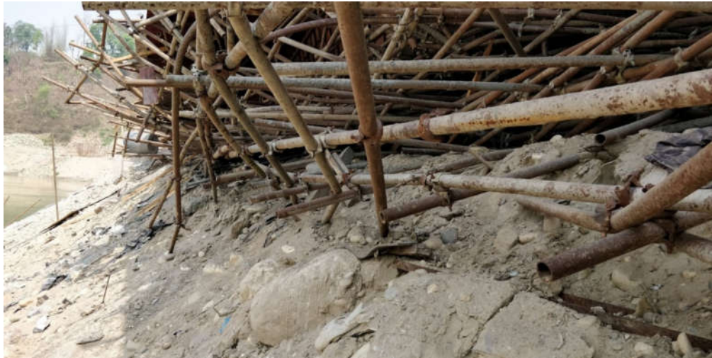
Figure 28. Settlement of downstream-most steel-section league-supporting falseworks.
