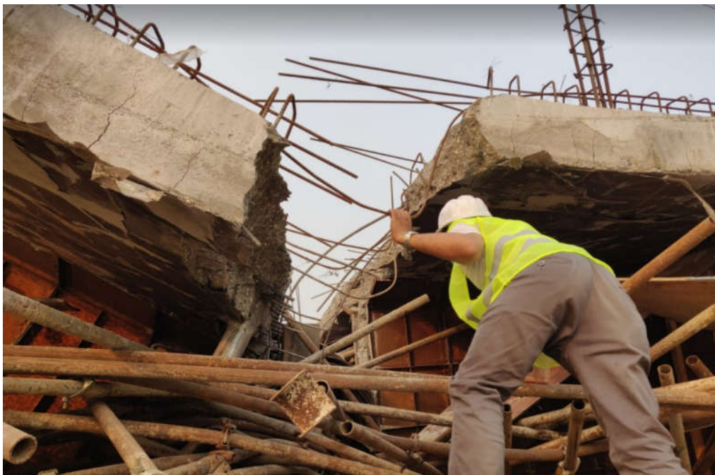
Figure 9. Fracture observed in slab of Span-2, including several flexural cracks near both sides of the main fracture region.
