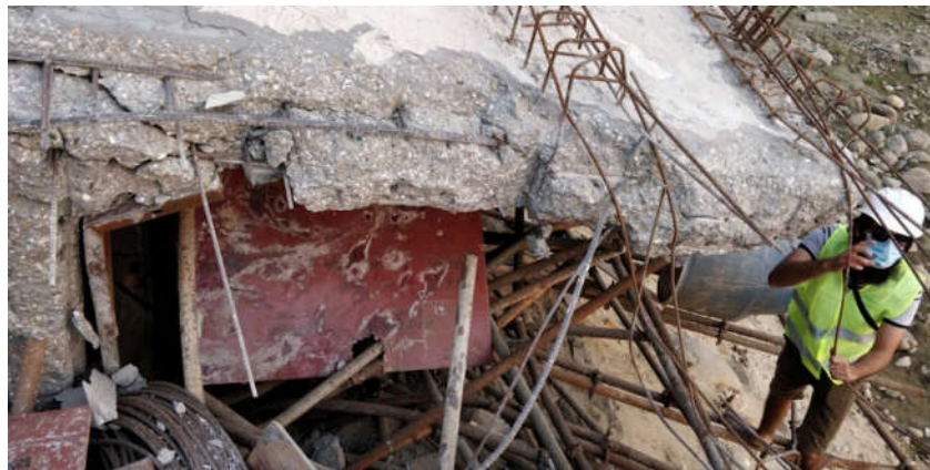
Figure 12. Pulled-out holes in slab in the fractured location.
