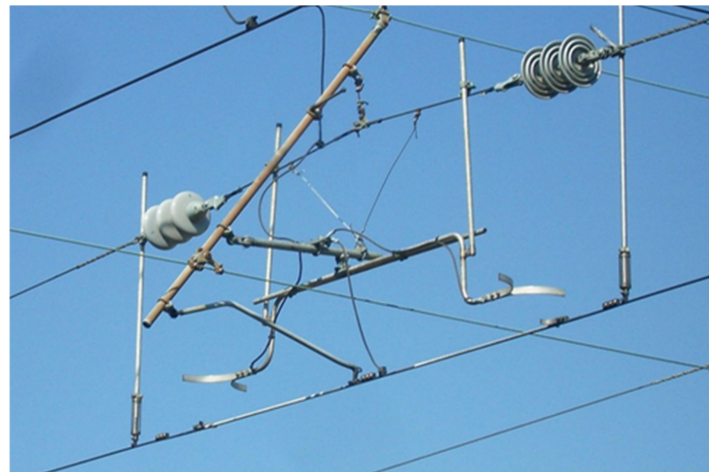
Figure 4. BR type 'skidless' ceramic bead neutral section installed in the line (photo Daniel Beardsmore).
