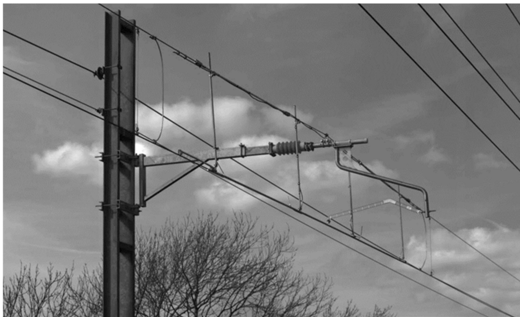
Figure 13. Neutral section installed at Melton (Old Dalby) from DBST trackside video [30].
