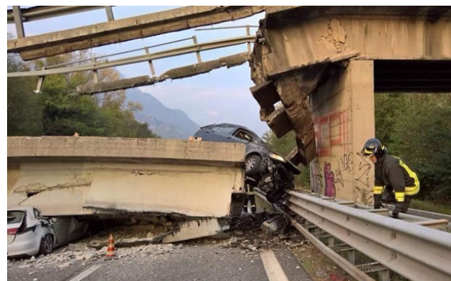
Figure 2. The Annone Brianza overpass collapse.
