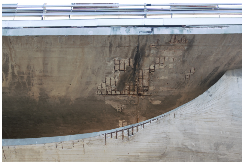
Figure 7. Deterioration of Gerber saddles and underlying vault.
