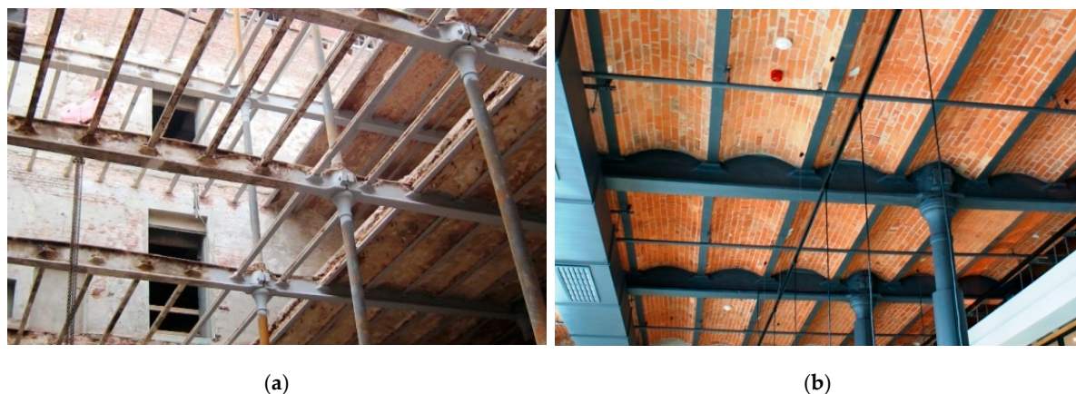
Figure 8. A cast-iron and steel structure of the former Poznański's spinning mill: (a) during and (b) after the completion of the restoration works.
