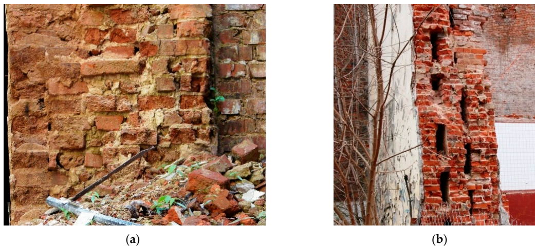
Figure 24. Examples of 19th century masonry walls: (a) careless workmanship, (b) hidden voids.
