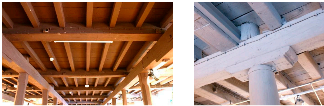
Figure 1. Wooden frame structure of the Ludwik Geyer's White Factory in Łódź—1837.
