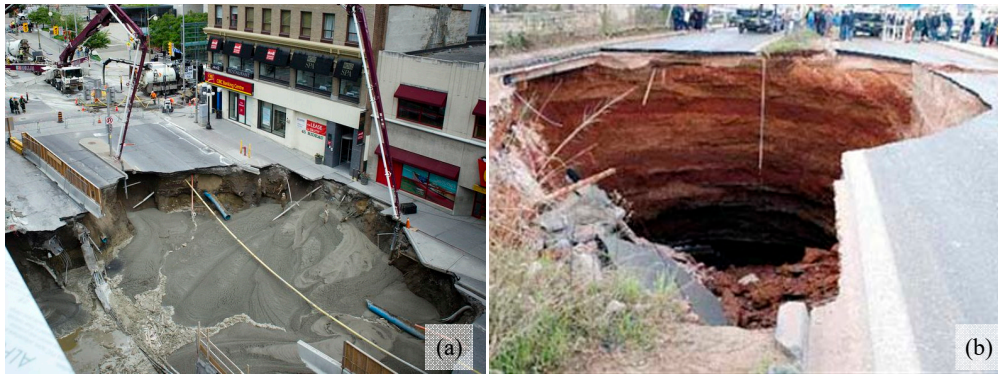
Figure 3. The problem of confidentiality in tunnel excavation data: (a) A sinkhole 8 m wide and 12 m deep opened up at the construction site of Ottawa’s light rail tunnel in 2016 [18]. (b) A 10 m wide and 15 m deep sinkhole opened up during tunneling beneath Doukissis Plakentias Ave., Athens for the Metro Line 3 in 2003 [19]. In both cases poor ground conditions have been reported but no other technical information is available.
