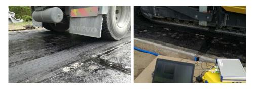
**Figure 10.** Monitoring of FBGs on the third day during the construction of top layer of the CyPaTs bicycle path at a temperature of 24 °C on the surface of the second base layer AC-10.
