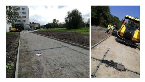
Figure 5. Installation of FBGs in the base asphalt layer directly on the base (first approach).
