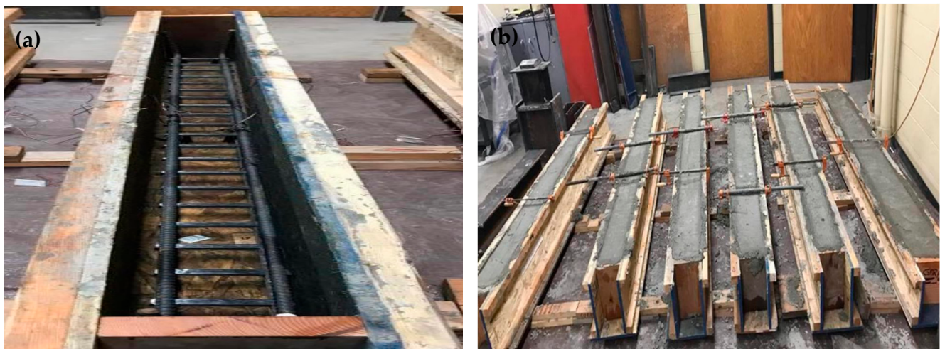
Figure 3. (a) Integrated arrangement of FRP and Conventional Steel Reinforcement within the formwork. (b) Casted concrete beams with clamps.
