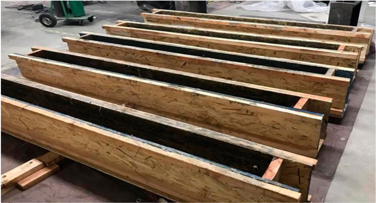
Figure 1. Prepared wooden formwork for concrete beams.
