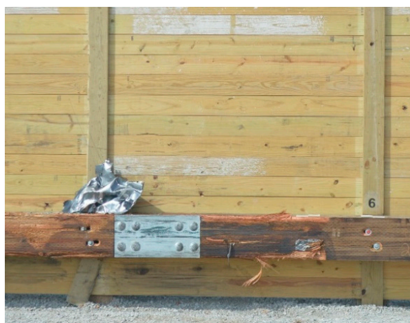
(b) System damage
